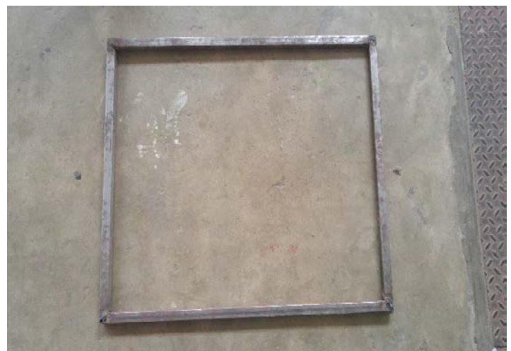
Fig. 6. Fabrication of upper frame
